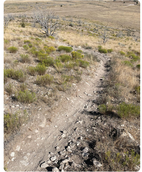
ObjID 86, Eastwood: Slope exceeds max recommendation.
