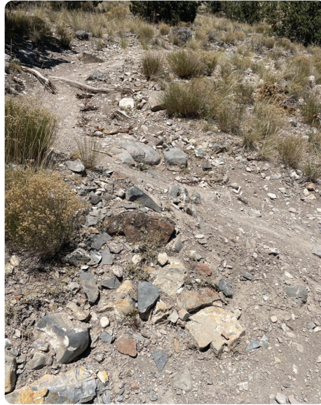
ObjID 25, Flintstone: Switchback Slope is too steep
