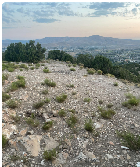
ObjID 45, Juniper Connector: While not on the main trail, this bridge is a major safety concern and if it is not repaired, it should be removed.
